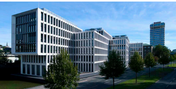
Overall view from the south/west
