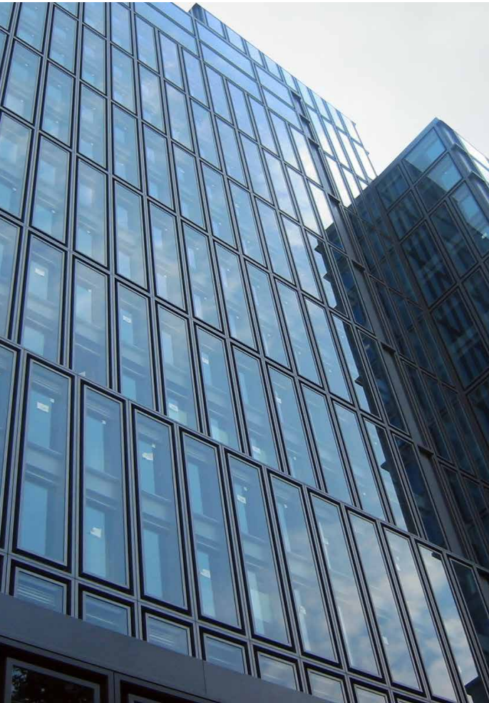
View of the west elevation
