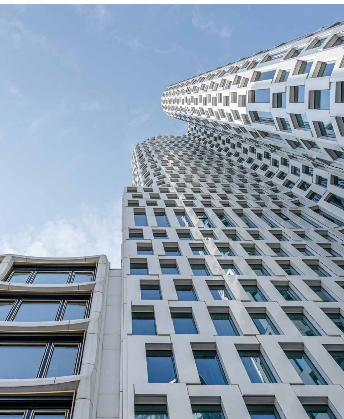
High- and low-rise building
