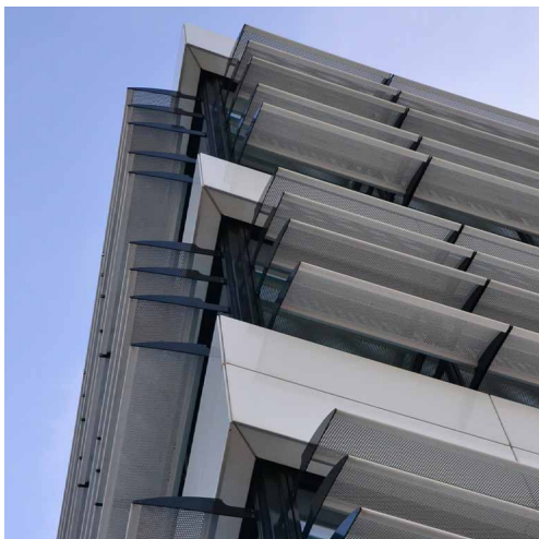
Building corner formation of low-rise buildings in construction unit A, B and C
