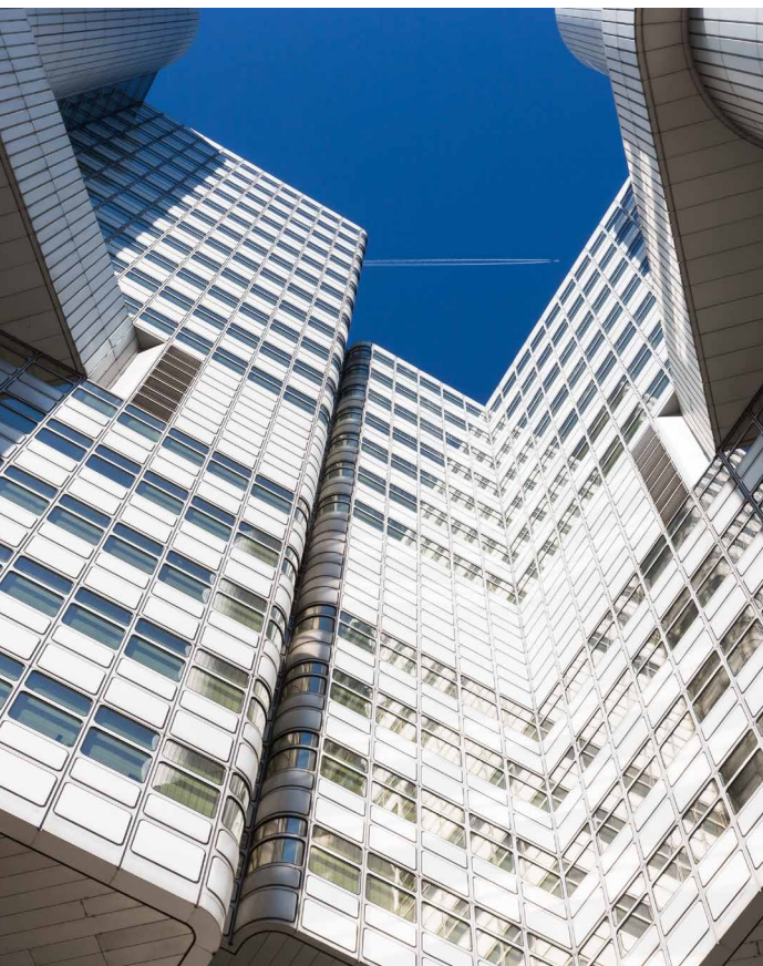
Detailed view of the refurbished façade
