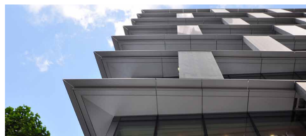
Overhanging sun blinds and concrete components on the new building
