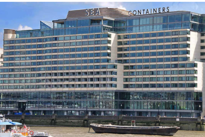
Core-renovated old building with erected rooftop bar - north view with Thames embankment
