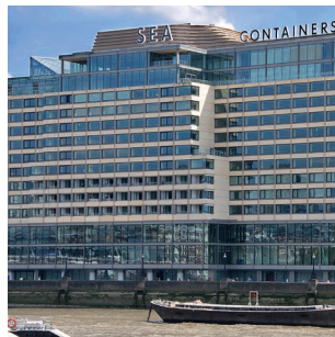
Sea Containers House, London
