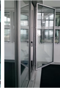
"Pop-in Window" - example of a vent parked at an angle
