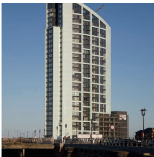
Alexandra Tower, Liverpool
