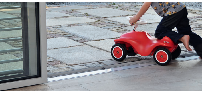
Barrier-free - height above FFL 15mm
