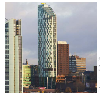
Tower West, Liverpool
